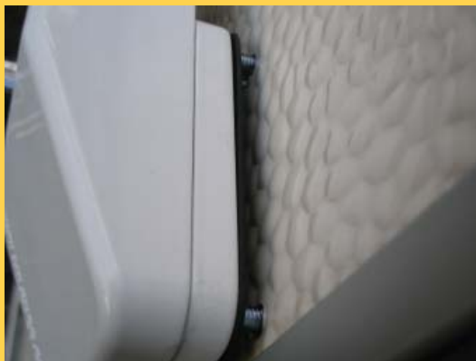
Mount and tighten 4 x M6 screws
