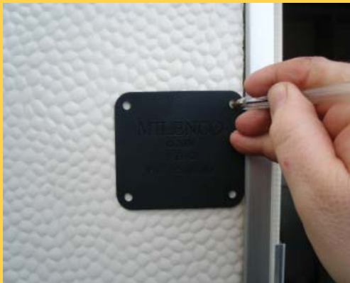
Use Gasket to mark drill position
