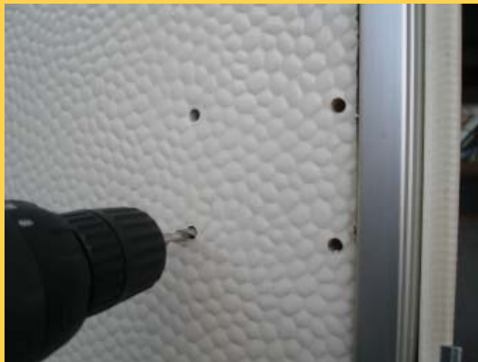
Drill 4 holes 7mm diameter
